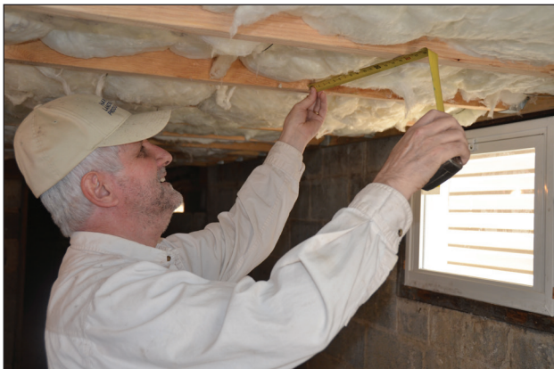
The Rev. Grant Spong hangs insulation in a basement.
